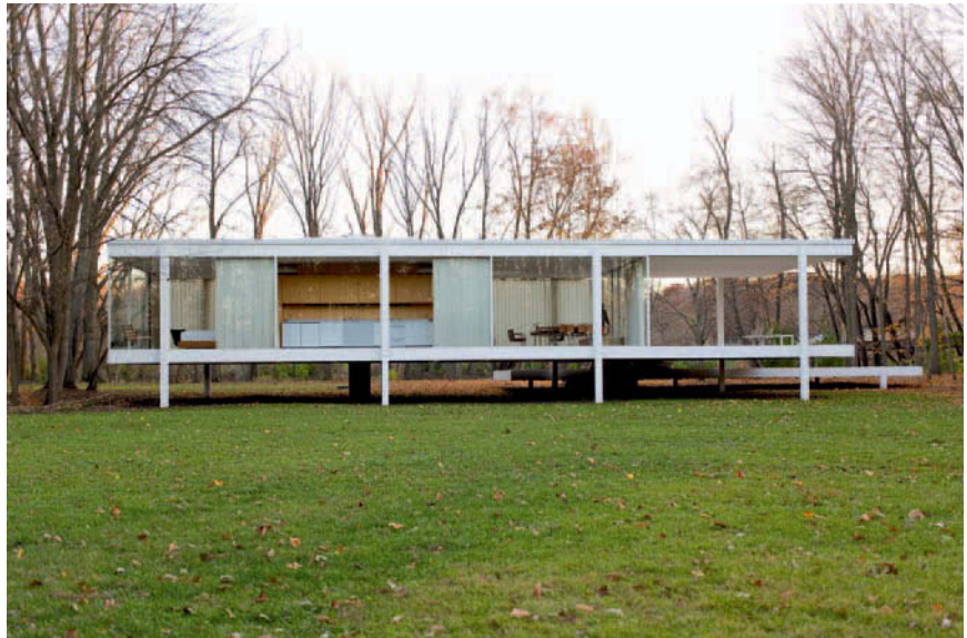
Figure 0.4 Farnsworth House, Illinois, 1951; Mies van der Rohe (1886–1969), architect. This building is supported by a rectilinear steel framework structure. The form is appropriate in the context of an industrialised society and for the span involved.
