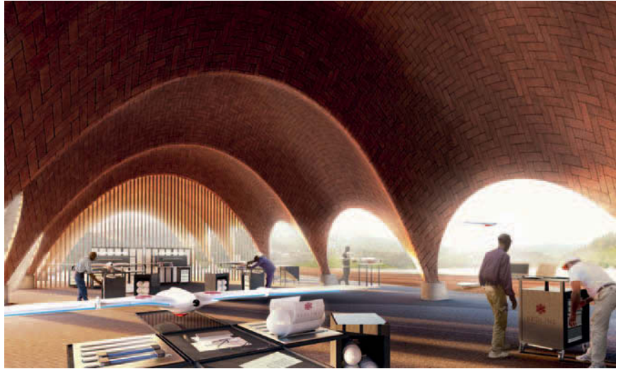
Figure 0.3 Droneport Prototype Building; Norman Foster Foundation, architects; Ochsendorf, De Jong and Block, engineers. The principal element of this building is a self-supporting (and therefore structural) multi-bay vaulted enclosure constructed from compressed earth bricks. Structural requirements have strongly influenced the choice of form and materials.
